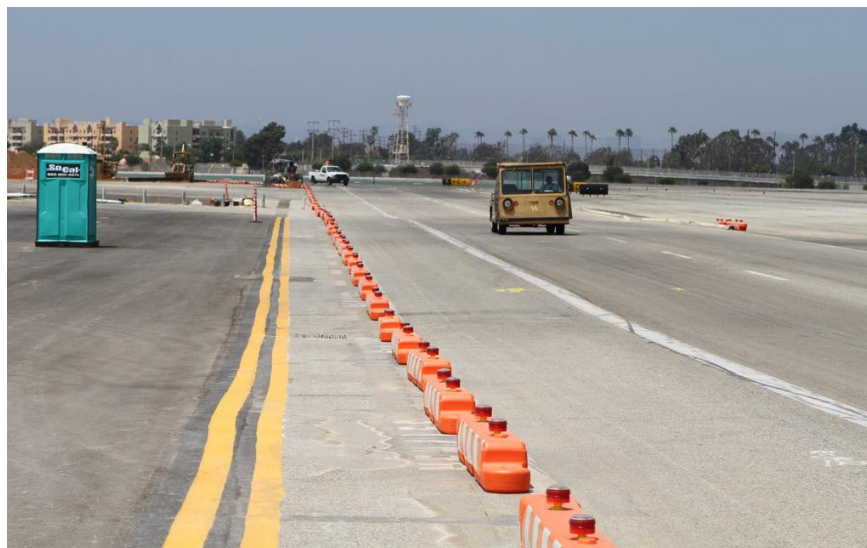
Figure 2. Low profile construction barricades provide a visual cue but may not prevent passage of pedestrians or vehicles (Source: OTW Safety, 2020).
